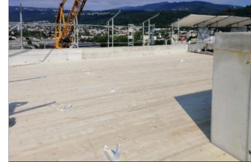
2019 Flat roof Biel, Switzerland, 200 m 2
