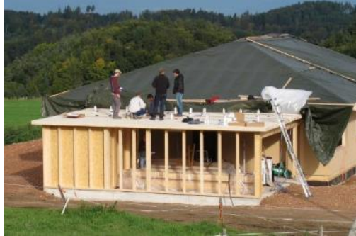
2013 Flat roof Carport, St. Antoni, Switzerland 54 m 2
