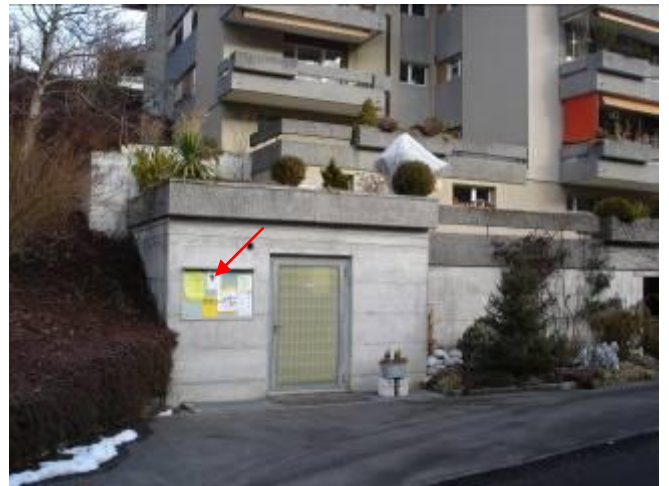
Bürgstrasse Nr. 23, BKW Trafostation
