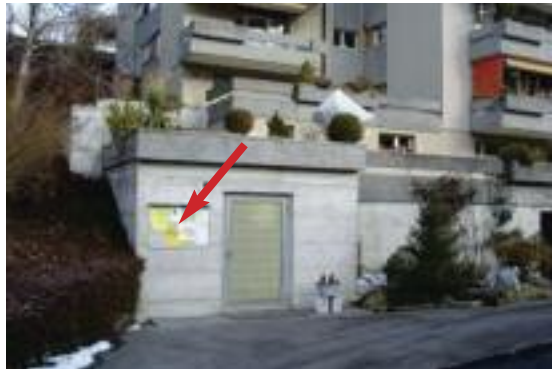
Bürgstrasse Nr. 23, BKW Trafostation
